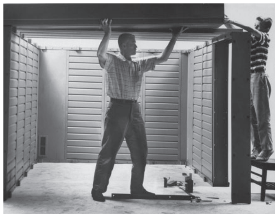
Fig 9. Art and Claude Carlson raise the roof on the family shelter. Shelter kits eased the burden of building a shelter from scratch. Life , 15 September 1961, p. 105. Photograph by Dimitri Kessel/Getty Images
